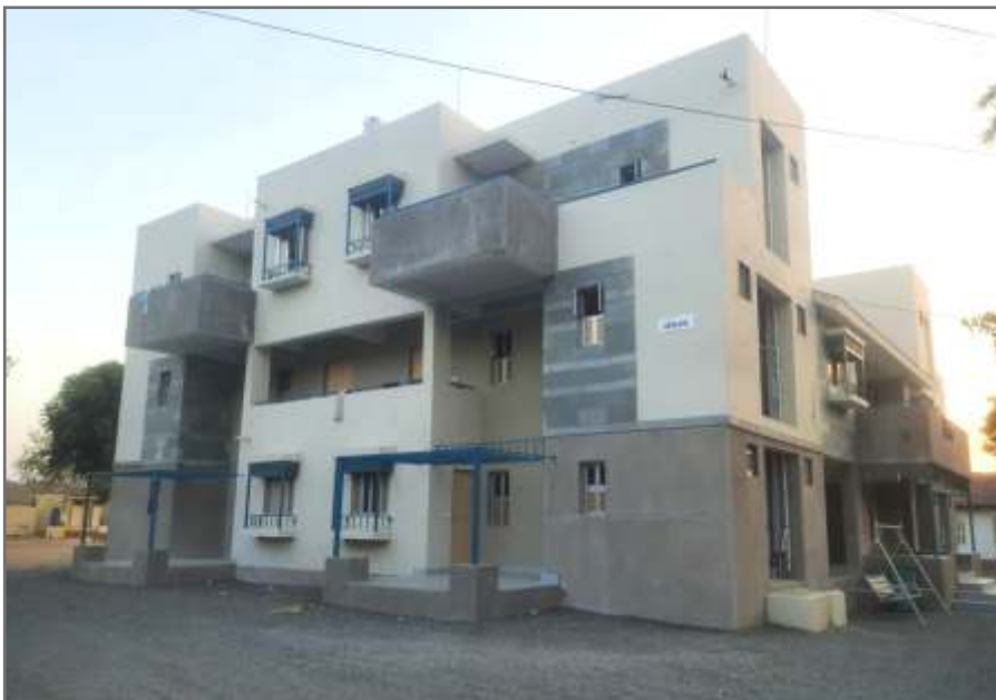
Picture 2: Construction of hostel facilities with the support of Pidilite
